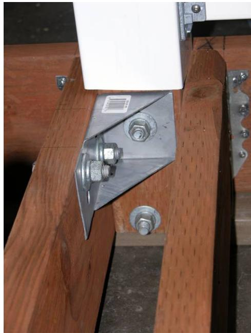
Between the posts was a vinyl top rail that contained an aluminum channel. Top rail height was constructed to be 36" above the deck surface. The vinyl bottom rail contained no aluminum reinforcement. Both rails were fastened to the posts with Stallion Fence Accessories brackets. Between the top and bottom rails, vinyl balusters were inserted into pre-routed holes that snugly accepted each baluster (Figure 2).
